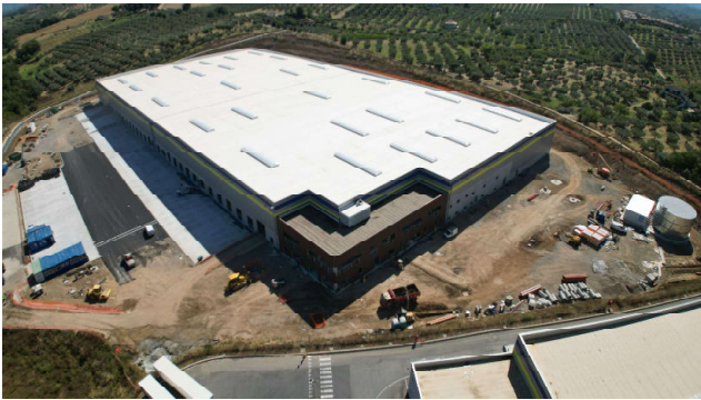
Poste Logistics AEW 3
